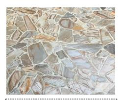
Example of well laid crazy paving. Joints are even with no long running uninterupted lines and no large mortar filled holes.
